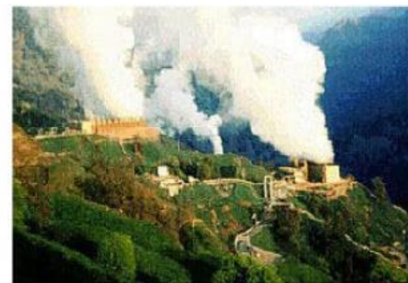
Geothermal Power Plant 地熱發電
