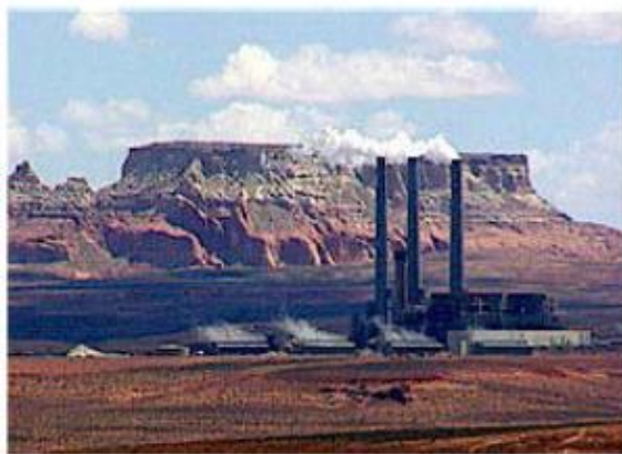
Fossil Fuel Power Plant 火力發電廠
