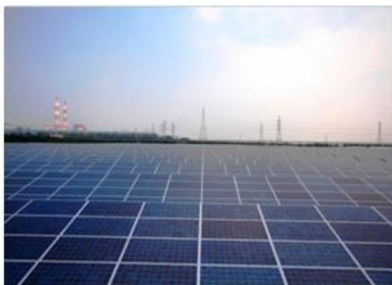
Photovoltaic Generation 太陽光電
