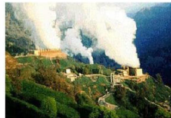
Geothermal Power Plant 地熱發電
