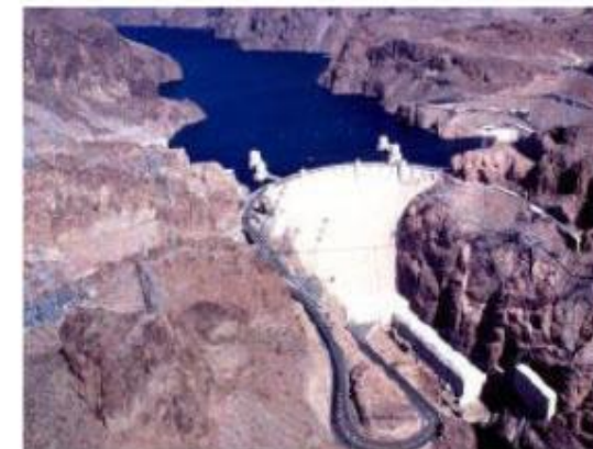
Hydroelectric Power Plant 水力發電廠
